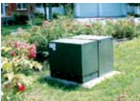
Pad-mounted transformer
