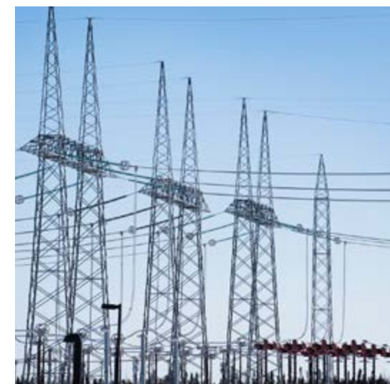
Radisson substation is a 735-kV converter substation and the starting point of the 450-kV direct-current interconnection line that runs from Baie-James to Sandy Pond substation, near Boston. Construction of the 1,500-km line began in the 1980s under a partnership between Hydro-Québec and New England's utilities. To date, the line has transported more than 100 billion kWh of clean electricity.
