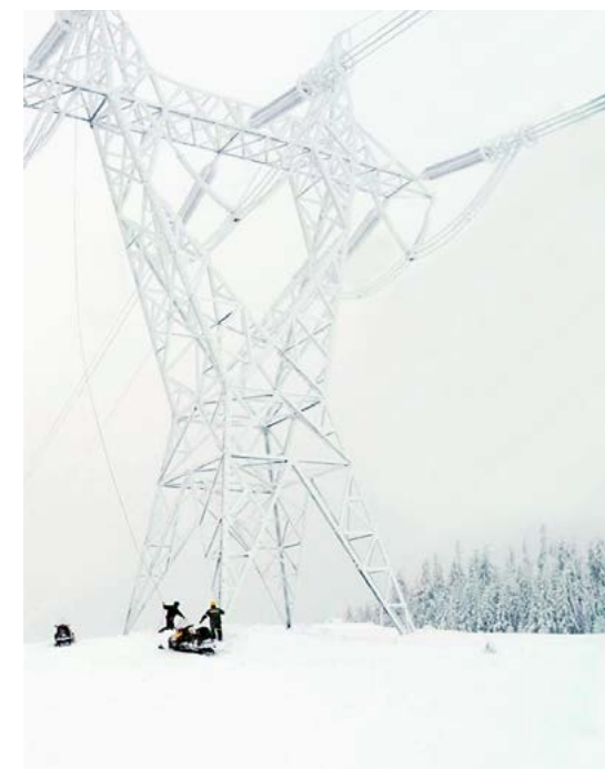
Ground-wire repair on the Saguenay-Jacques-Cartier line.
