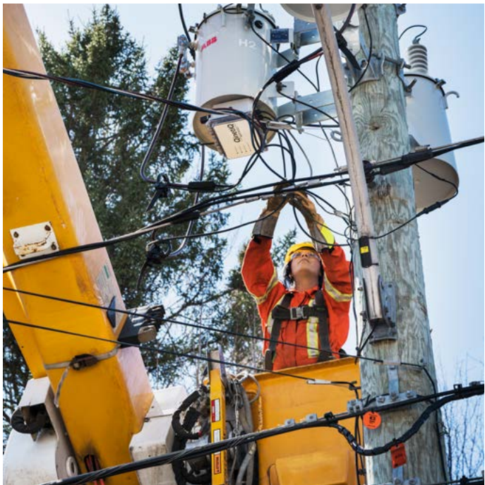
Installation of the MILE intelligent power-line maintenance system on a distribution line in the Laurentides region.
