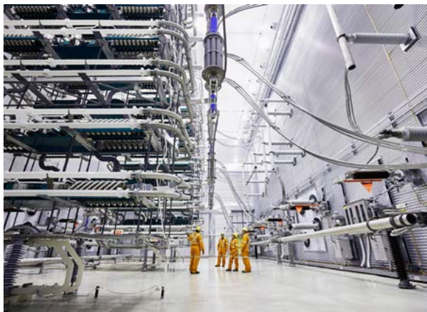
Converter room at Outaouais substation, which allows interchanges with Ontario.
