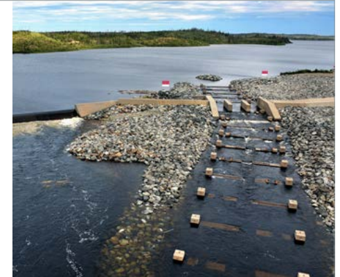
The fish pass built on the Eastmain at kilometre point 207—one of several fish protection measures.
