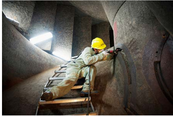
Powerhouse mechanic Carl Lalande carries out maintenance work on a generating unit at Carillon generating station, in the Laurentides.
